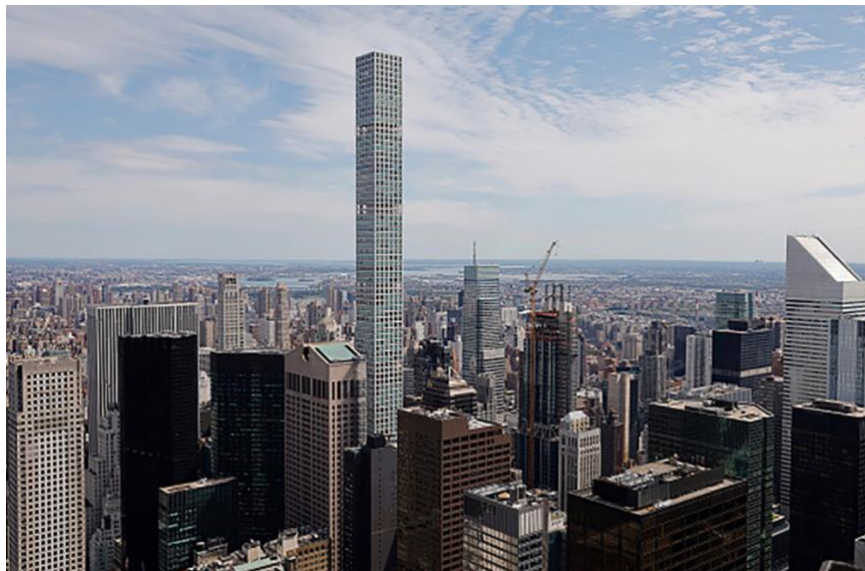
A view of Park Avenue shows 425 Park while it was under construction.
